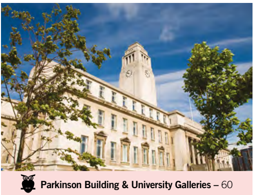
Parkinson Building & University Galleries – 60
