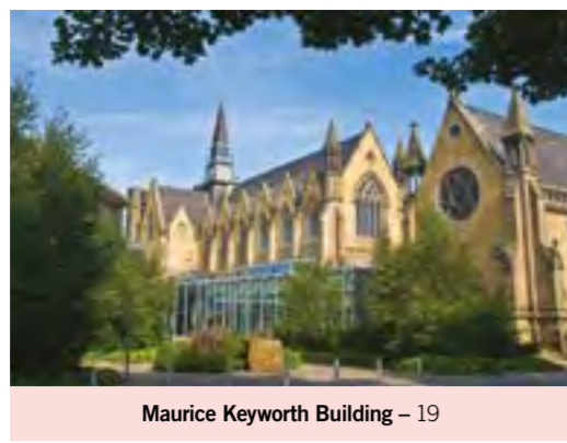
Maurice Keyworth Building - 19
